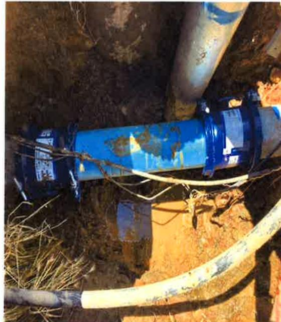
*Main break before and after pictures Replaced 30"x6" water main on Spinnaker*
