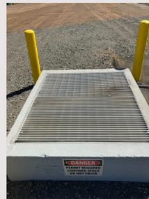
2) Ladder guard installed to secure the access due to it being a permit required entry also known as confined space.
