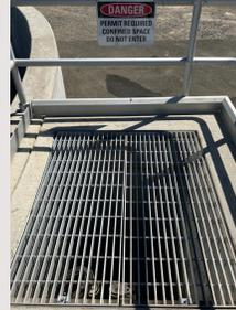
1) Scum Box-restraints added to grate to secure entrance and labeled as a permit required entry (confined space )
